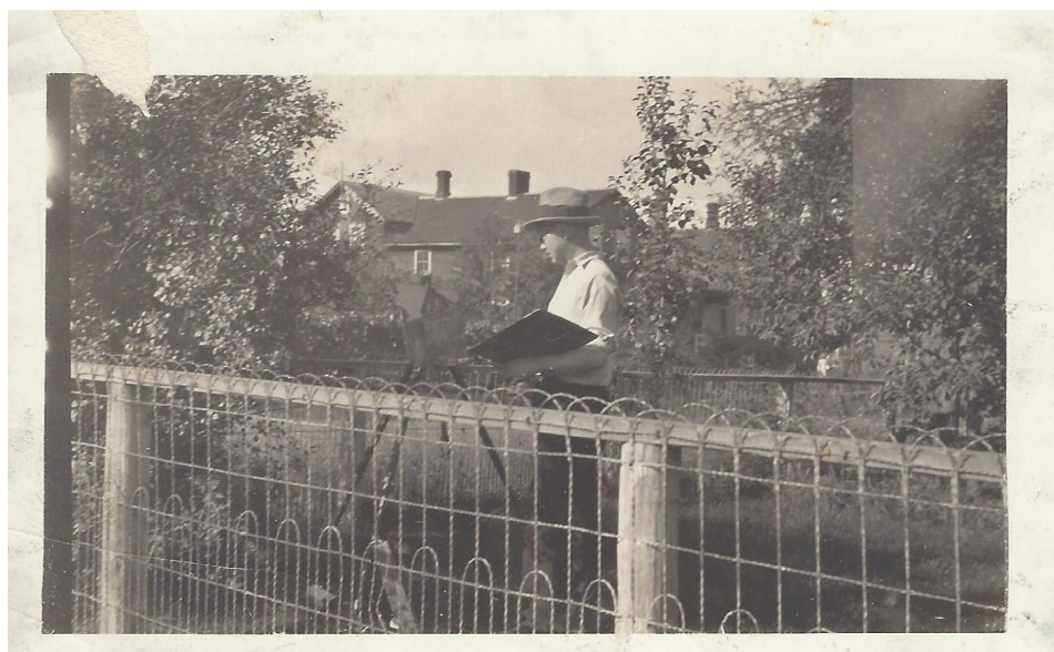
Wood fence frame with attached wire fencing (round fence posts)
